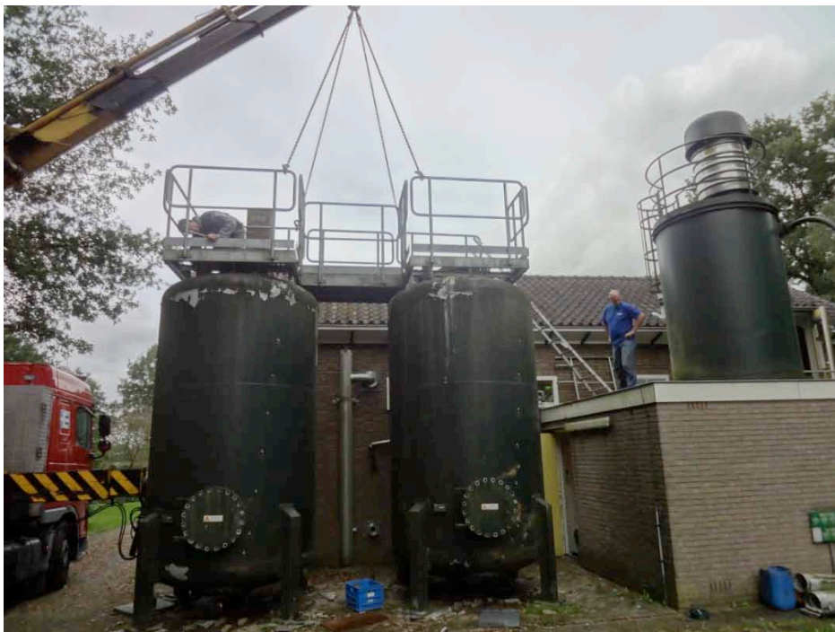
Demontage ps Elburg
